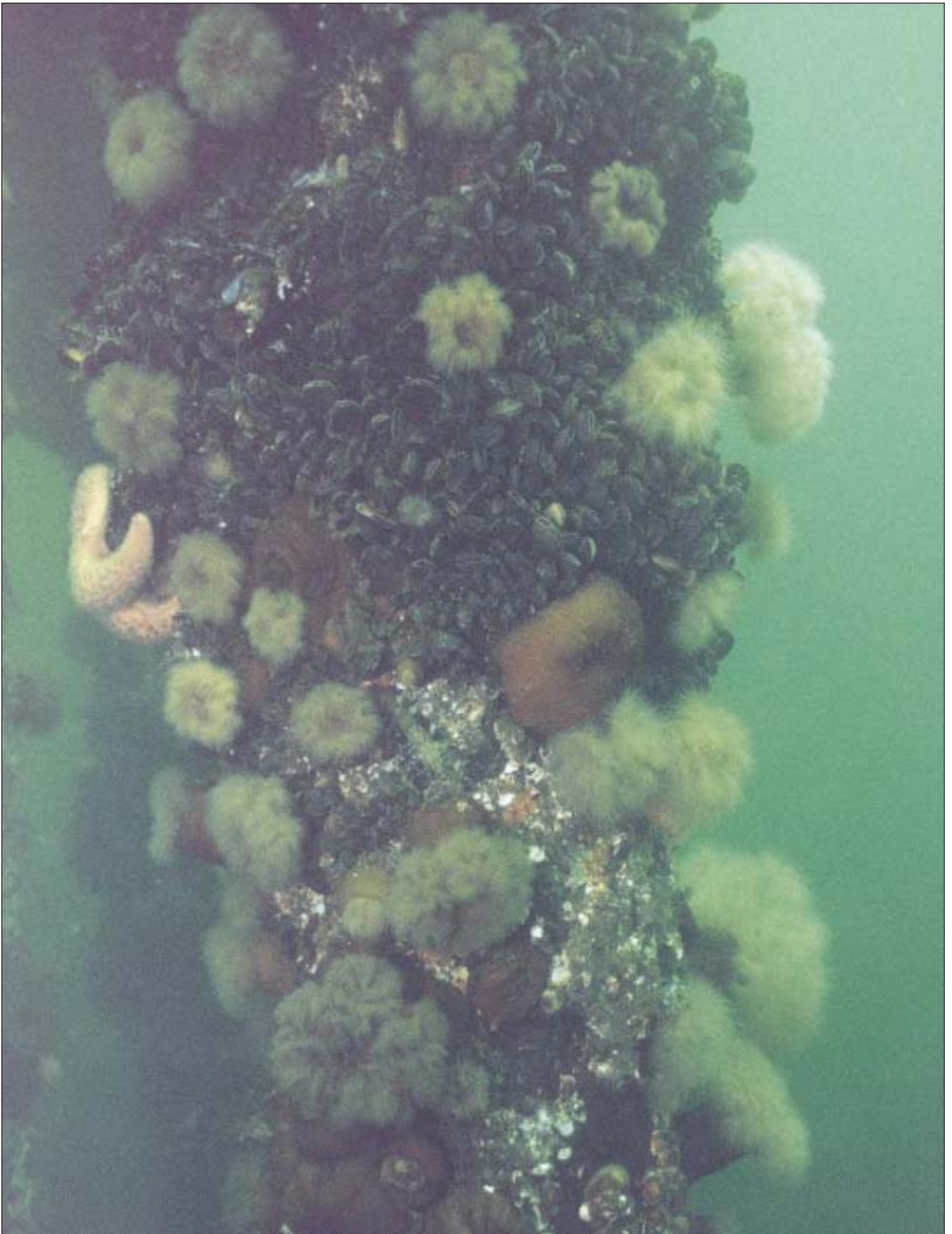
Invertebrate community growing on a new creosote-treated marine piling in Sooke Basin
